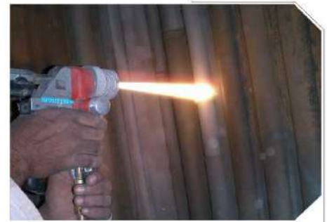
ANTI-EROSION & ANTI-CORROSION COATING ON BOILER TUBES
